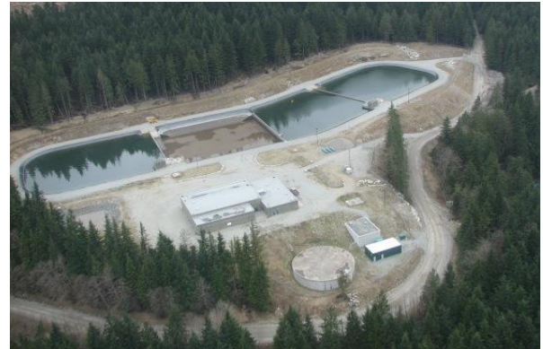
Norrish Creek Water Treatment Plant
