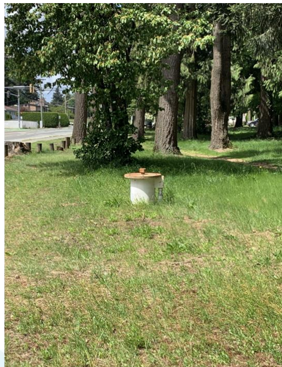
Bevan Wellfield - Groundwater Source
