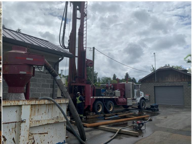
Farmer 1 - Well Rehabilitation (Re-Development) using Water Jetting
