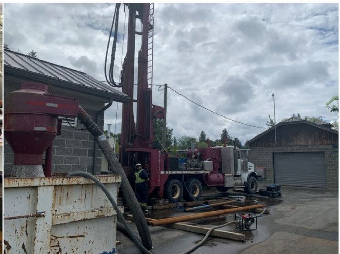
Farmer 1 - Well Rehabilitation (Re-Development) using Water Jetting
