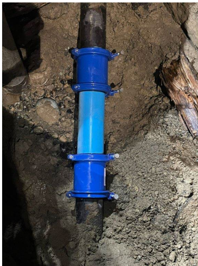
WATER MAIN – 150 MM DIAMETER, The water main is exposed following the repair of a leak in 2024 (South Fraser Way).
