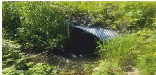
Photo 5: Downstream at Downes Creek May 31, 2022
