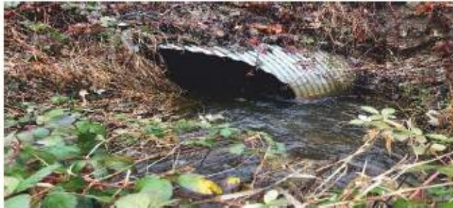
Photo 7: Downstream at Downes Creek Jan 13, 2023
