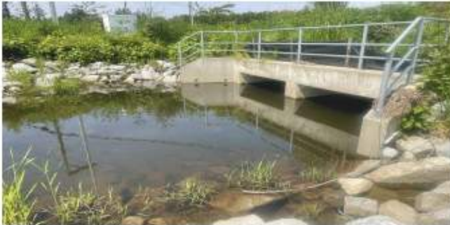
Photo 1: Upstream at Fishtrap Creek May 31, 2022
