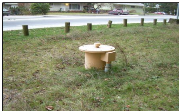
Groundwater Well Head
