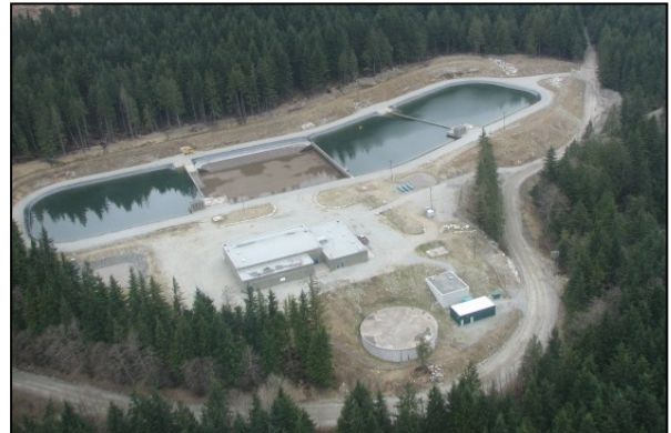
Norrish Creek Water Treatment Plant
